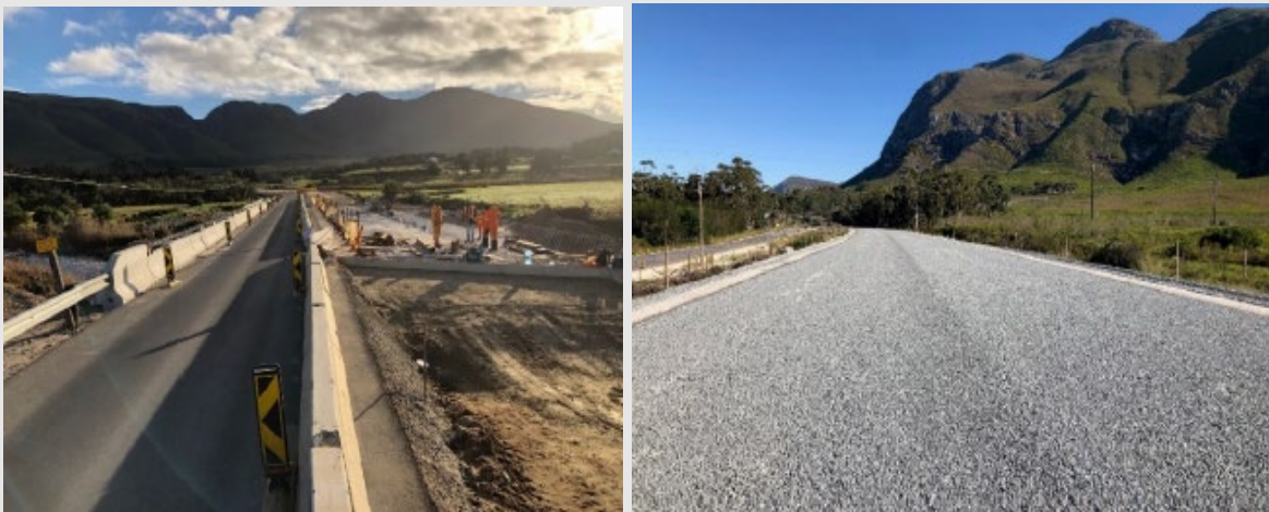
Photo: Rehabilitation of TR02802 between Hermanus & Stanford (Overstrand Municipality), OPMII 2021.
