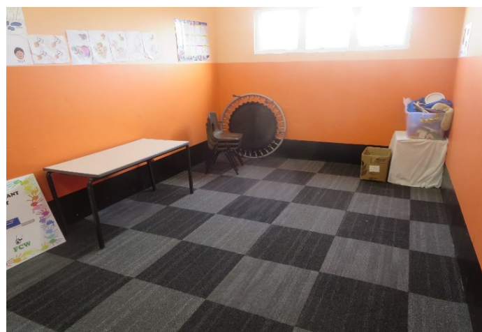
New Flooring at Nomaxibiso ECD Facility (City of Cape Town)
