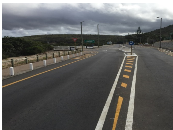
Roadworks on MR00332 between N2 and Still Bay (Hessequa Municipality)
