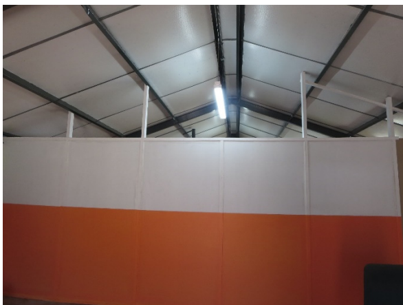
Classroom Partitioning at Goldy Locks ECD Facility (Witzenberg Municipality)
