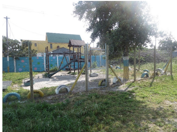
Security Fencing at Siyakhanyisa ECD Facility (City of Cape Town)
