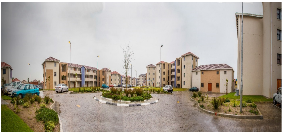
Scottsdene Rental Estate, Social Housing Project (City of Cape Town)
