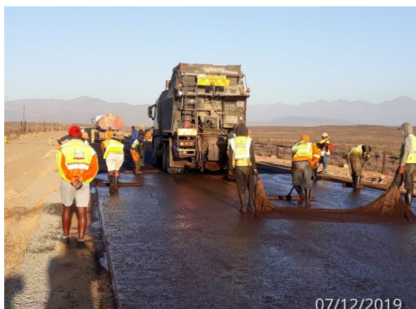
Roadworks from Calitzdorp to Calitzdorp Spa (Kannaland Municipality)
