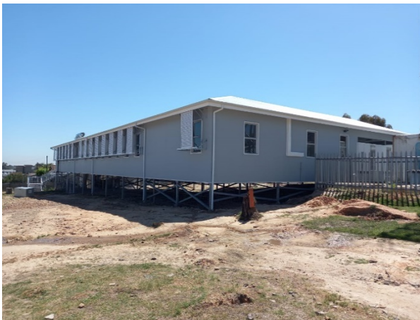
Sonstraal Hospital (Praal) – Intermediate Care Ward
