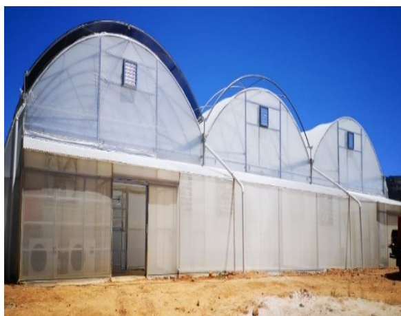
Tunnels for plant propagation
