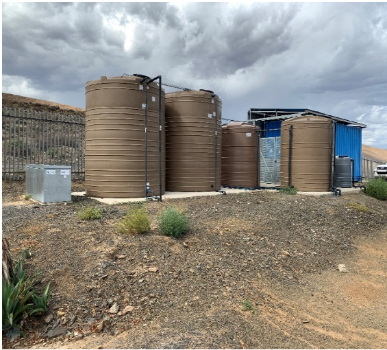
Water resilience - Laingsburg Hospital
